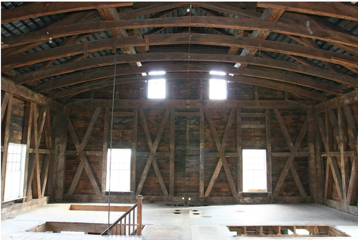
Exposed Timber Frame Walls after removal of Interior Apartments
