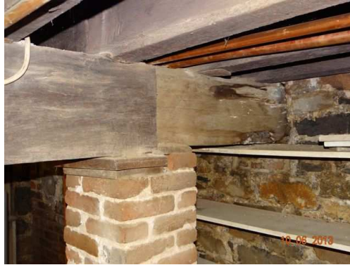
Main basement support beam with replaced end and newer support column
