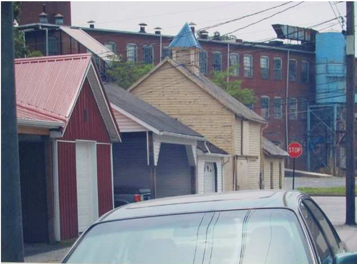
The garage as it exists today in the alley behind Walnut Street. Photo courtesy of Jack Fisher.
