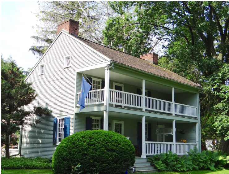
125 Stein Lane, north side
