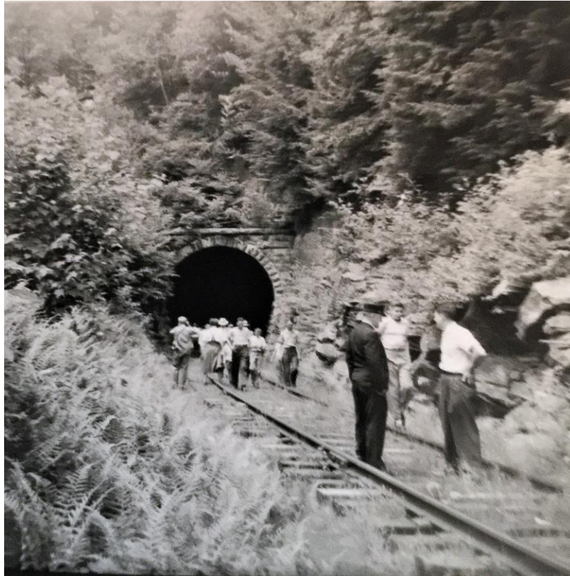
East End of Paddy Mountain Tunnel
