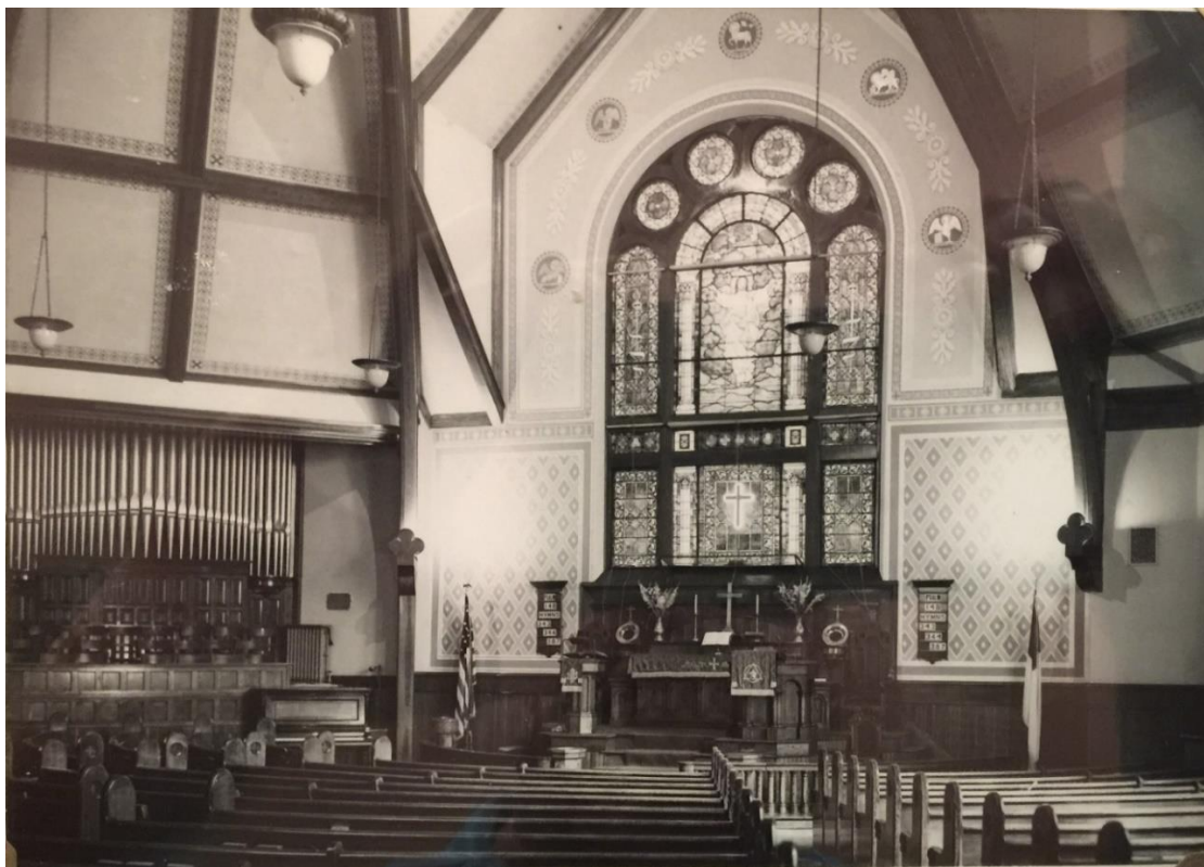
Interior of 1902 church showing original pipe façade of the Felgemaker Organ
