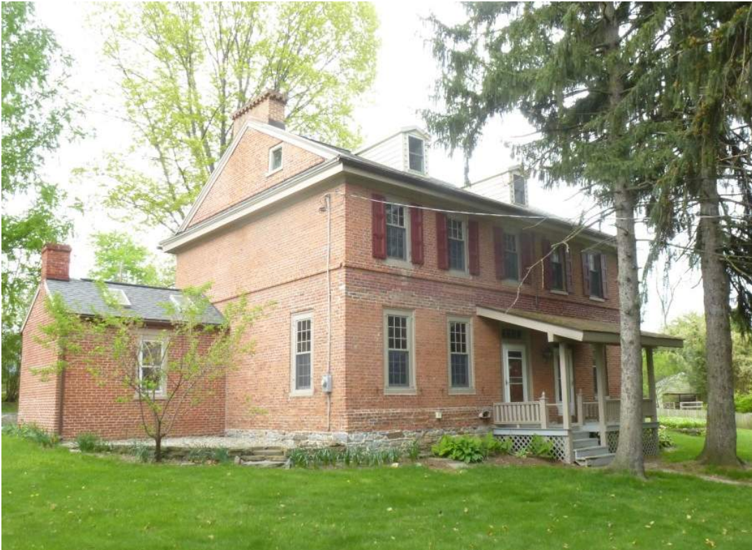
Figure 6 Robert Barber house near Wright's Ferry, Lancaster County, b. 1760, showing evidence of removed pent roof.
