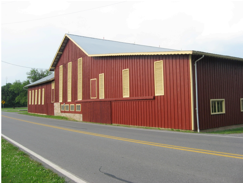
Manbeck Barn in 2012 after renovations
