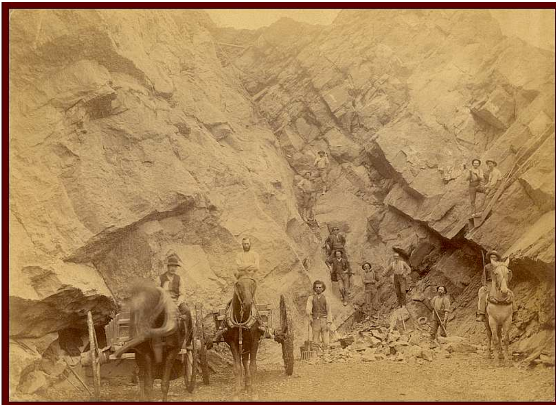
Limestone Quarry near Winfield
