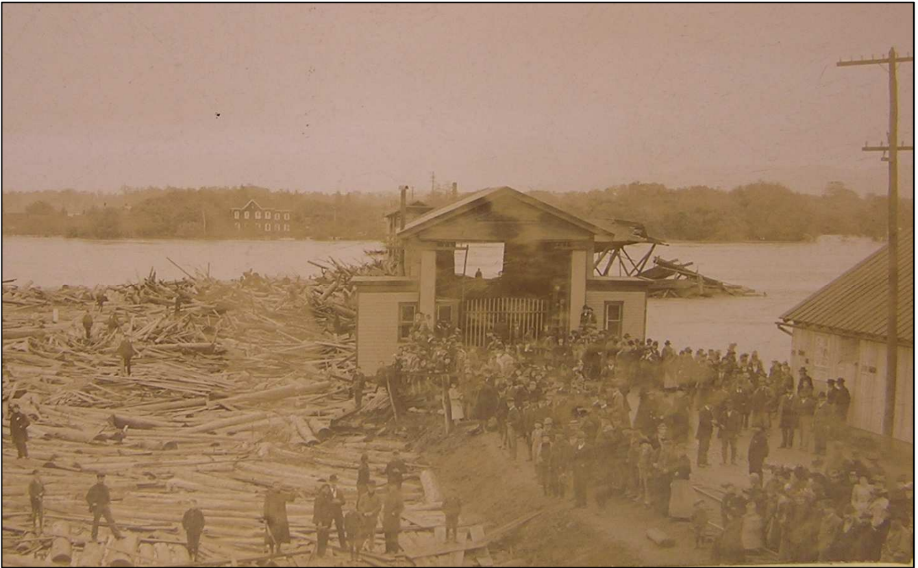
The flood of 1889 destroyed the bridge over the Susquehanna at Lewisburg.
