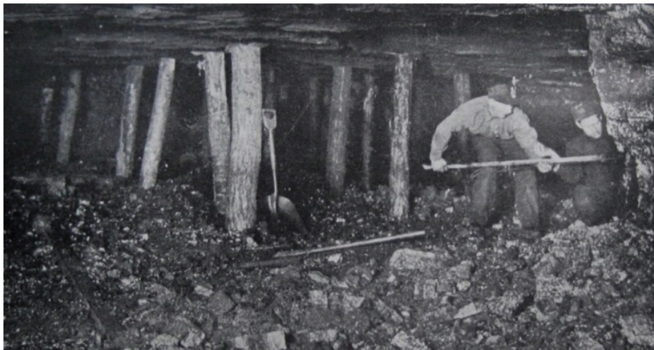
Taken in 1900 at the Lackawanna Colliery in Lackawanna, PA, this photo shows the use of props to hold up the rock ceiling as miners work to remove the narrow vein of coal. Photo: Public Domain
