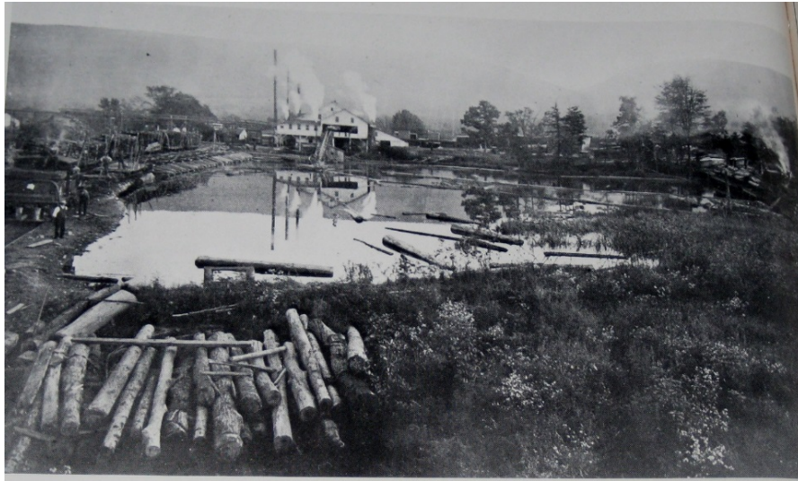
Laurelton Mill at Laurel Park. Logs were delivered by narrow gauge rail (left and right) to the mill pond to await sawing. They were individually pulled up the ramp (center) into the mill. Sawn lumber was collected in huge stacks to the right of the mill; the Lewisburg and Tyrone Rail Road hauled the lumber to destinations beyond. Photo: Public Domain
