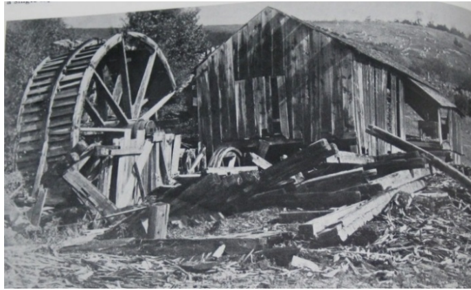
Few photos exist of water powered sawmills. This one was taken circa 1890 in Potter County of the remains of a typical early, family-operated small mill. Photo: Public Domain.
