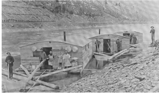
Three Arks for a log drive on Pine Creek, in Lycoming or Tioga County, Pennsylvania, USA. The left ark was for cooking and dining, the middle ark was the sleeping quarters, and the right ark was for the horses. The arks were built for just one log drive and then sold for their lumber. The line of the Jersey Shore, Pine Creek and Buffalo Railway can be seen on the eastern shore, and the mountainside behind it is nearly bare of trees from clearcutting. Photo: UCHS
