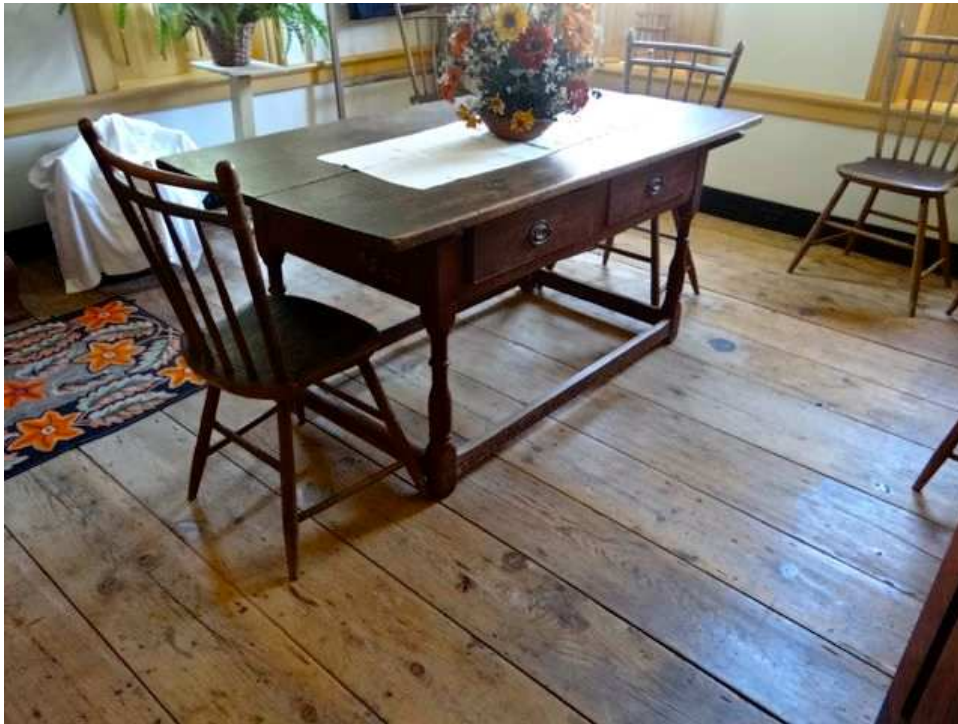
Example of original, unfinished floors
