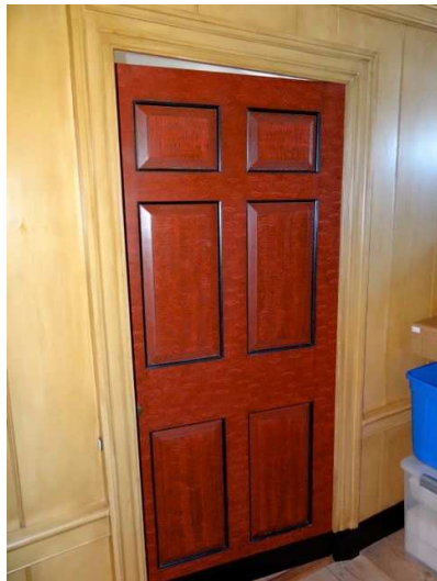
Paneled doors from downstairs were restored to their positions and given painted graining
