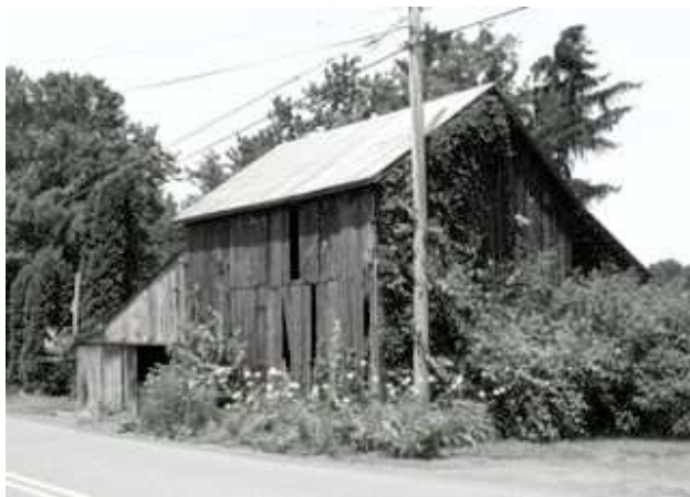
c. Two-bay frame ground barn south of Winfield
