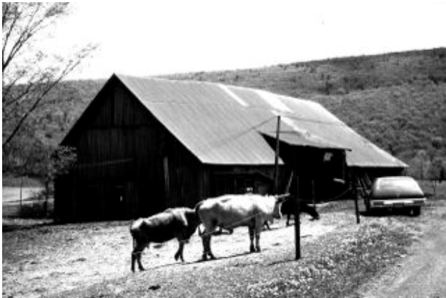
c. Double-crib ground barn near White Spring
