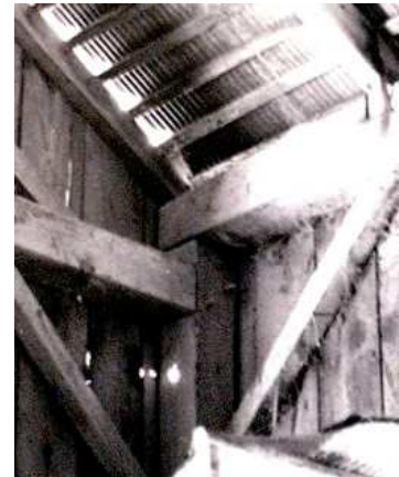
c. Mortise joint at tie beam
