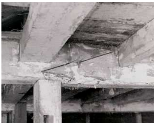
a. Scarf joint at summer beam
