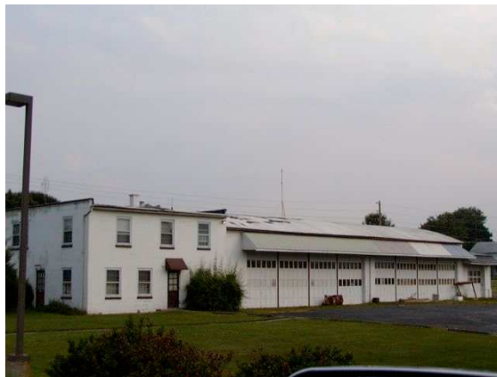
Hangar #1 shortly before it was razed in 2003. (Courtesy of Melvin Reed)
