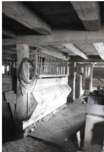
b. Feeding aisle and horse stalls
