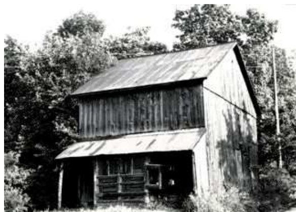
d. One-bay frame ground barn south of Furnace Road
