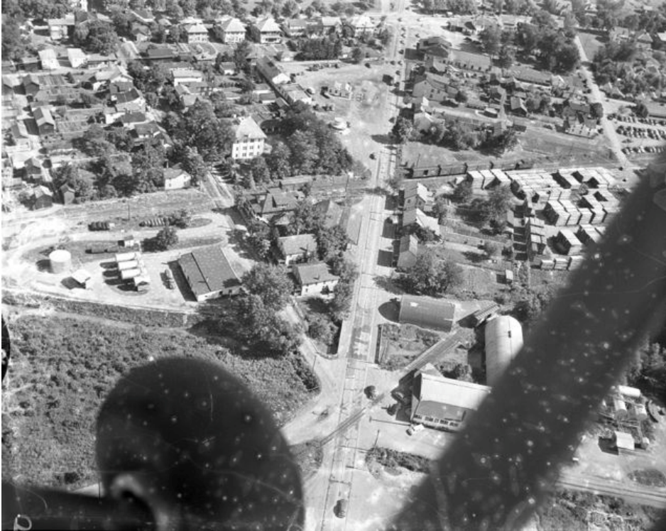
Recreational fliers used the Lewisburg Airport for flights to photograph Lewisburg and the surrounding areas from the aircraft. This aerial view of Lewisburg shows Route 15 (top to bottom in the center). To the right, stacks of wood lie at the Pennsylvania House property near the railroad line. At the upper left, one can identify a three-story apartment building that once was the West Ward School. (Courtesy of the Union County Historical Society)
